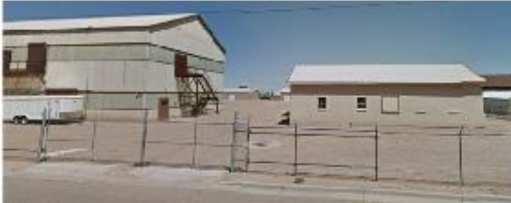
Figure 26: Site I - 310 E. Washington St. (Google Image 2012)
