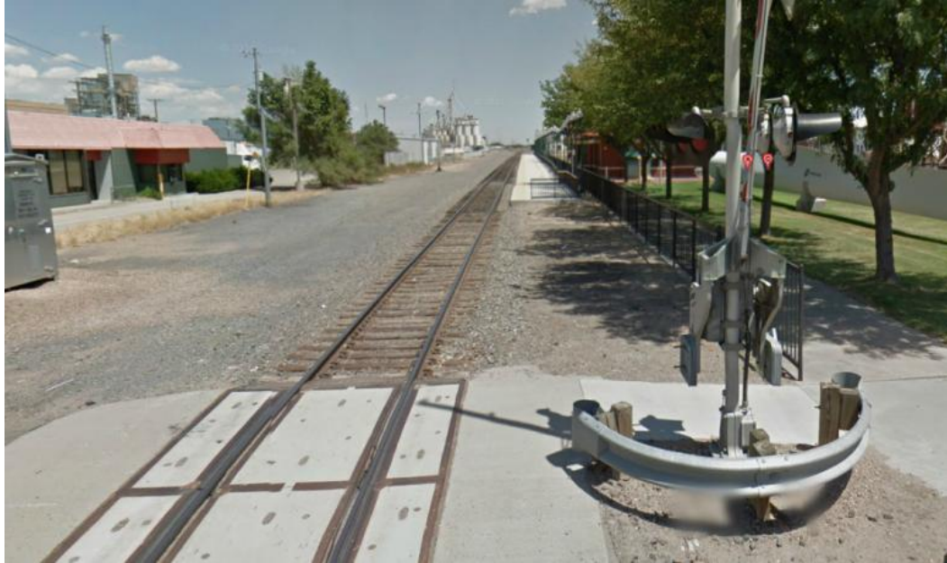
Figure 50: Railroad tracks with gravel on each side (Google Image 2012)
