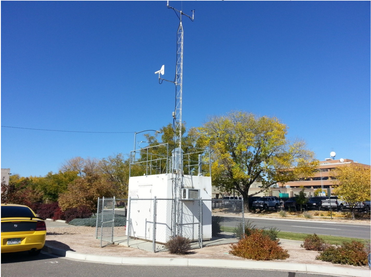
Site Photo: Shelter and inlets (looking NORTHWEST )
